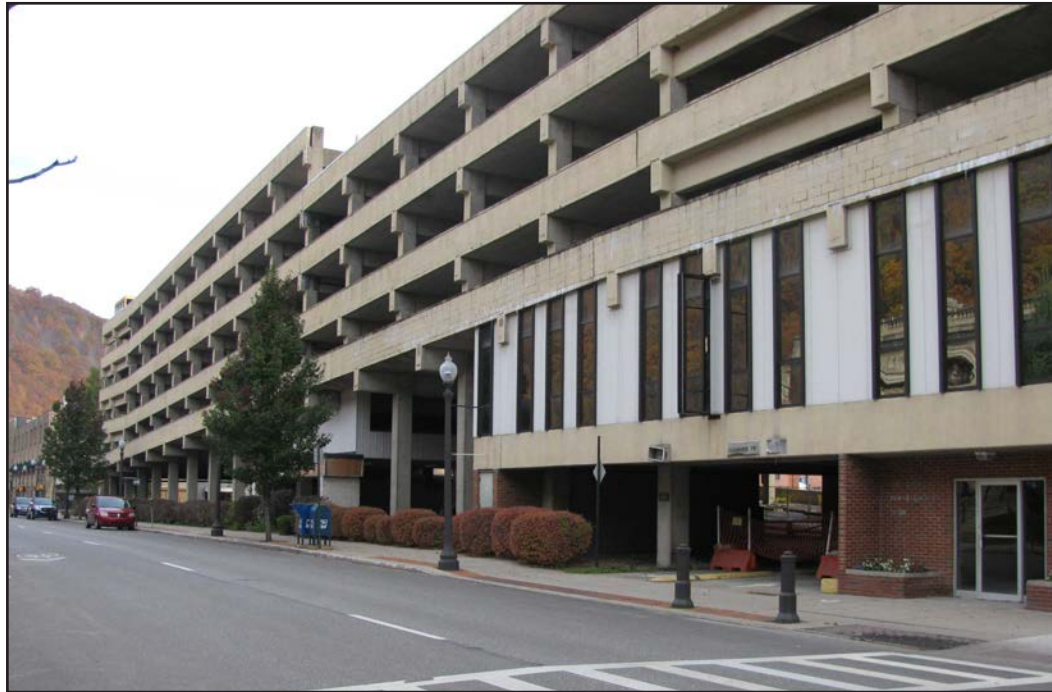
The Oil City parking garage currently sits empty and condemned on 1-acre of space within the Northside Business District.
